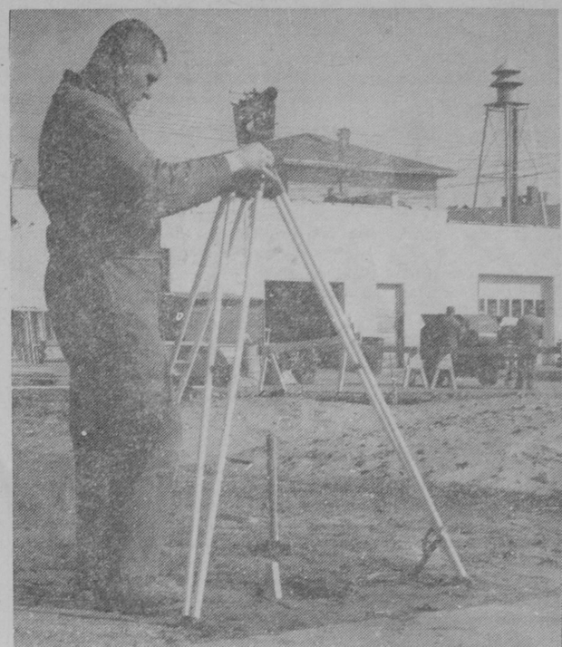
Construction on East Tawas City Hall Stopped
