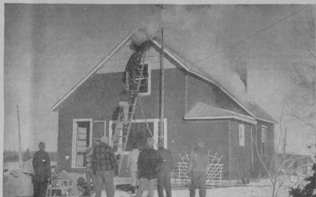
SMOKE POURS from the Grant Bessey residence on Townline Road Sunday morning. Tawas City firemen battled the blaze for about three-quarters of an hour before bringing it under control. Fire damage to the roof, water and smoke damage to the upper portion was considerable. There was very little damage to the lower portion of the building, however. Downstairs furniture was saved by the Besseys, with the assistance of neighbors.—Tawas Herald Photo.
