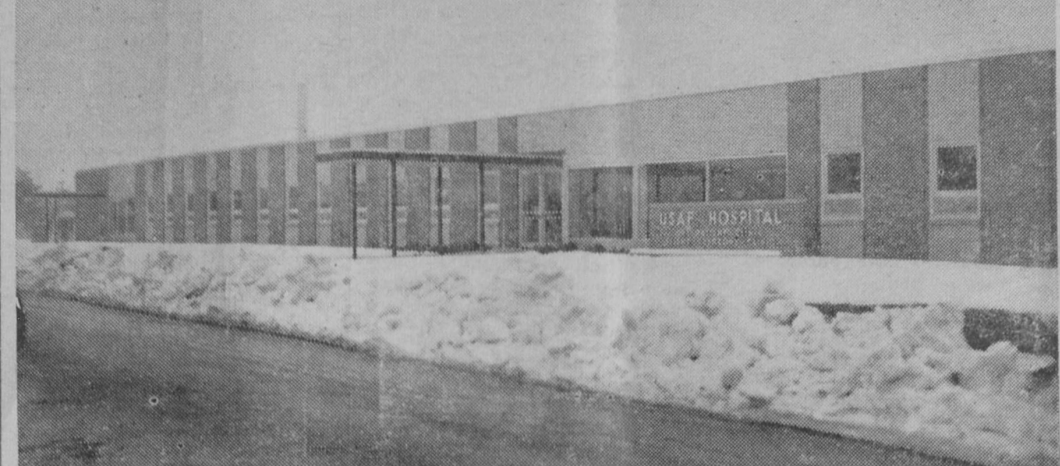
Contractors are adding finishing touches and installing medical facilities in the new hospital.
