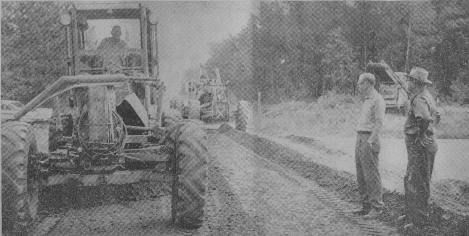
WATCHING these graders mix "batter" for a new method of road construction are Joseph Kelly of Bituminous Materials Company, Bay City, and Rudolph Anderson, right, general foreman for the Iosco County Road Commission. New techniques are being used to surface Bissonette Road west of Oscoda. Another picture showing work is printed on page 8.—Tawas Herald Photo.
