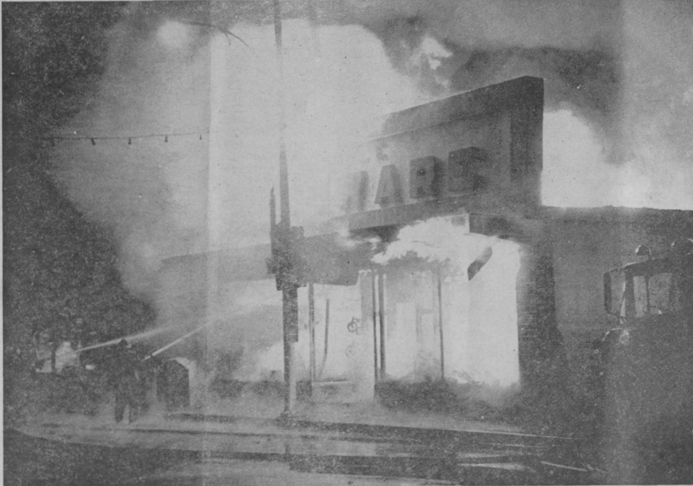
SMOKE AND FLAMES pour out of two Tawas City stores during the height of last Thursday morning's fire. Completely demolished was Tuttle's Hardware on the right, while Whitfield's Department Store was gutted. Firemen from three departments fought the
