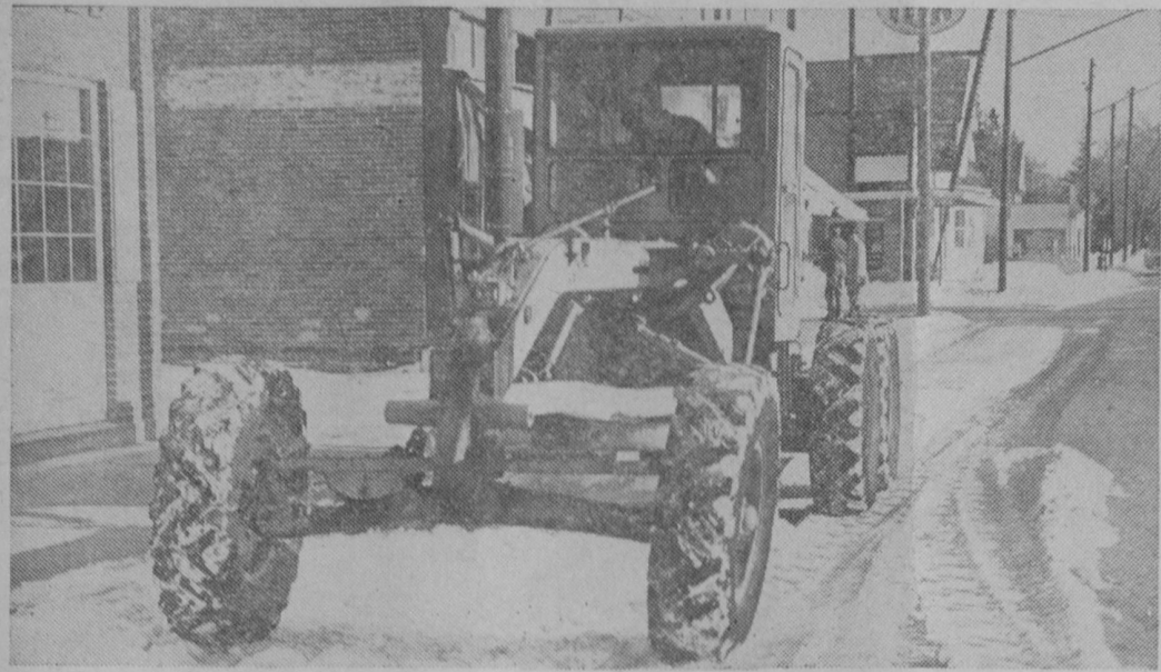
AIDING CREWS in digging out Tawas City streets following recent snow storms has been this grader, recently purchased from the United States Forestry Department. The unit became surplus upon its replacement and the city purchased it for street construction work.—Tawas Herald Photo.
