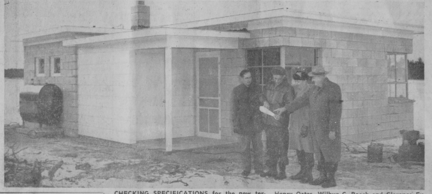
CHECKING SPECIFICATIONS for the new terminal at Iosco County Airport prior to acceptance Saturday are, left to right, Edward Seifert Jr., Henry Oates, Wilbur C. Roach and Clarence Everett. The building was constructed by Huron Development Company.—Tawas Herald Photo.
