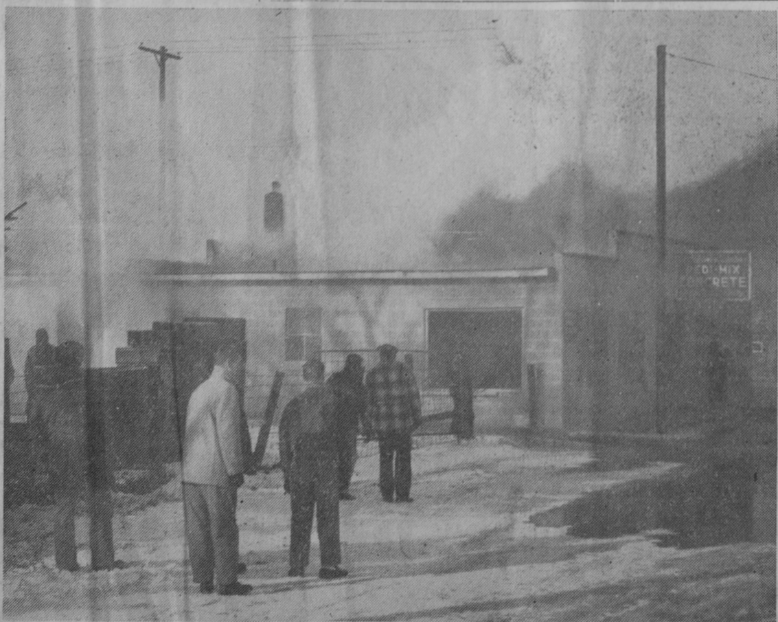
SMOKE POURS from City Fuel and Mason Supply, East Tawas, Friday after an exploding gas tank set the building on fire. Volunteer firemen
