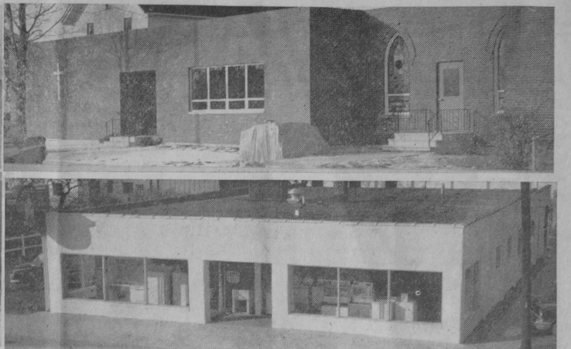
New Zion Lutheran School at top; remodeled Consumers Power Building below
