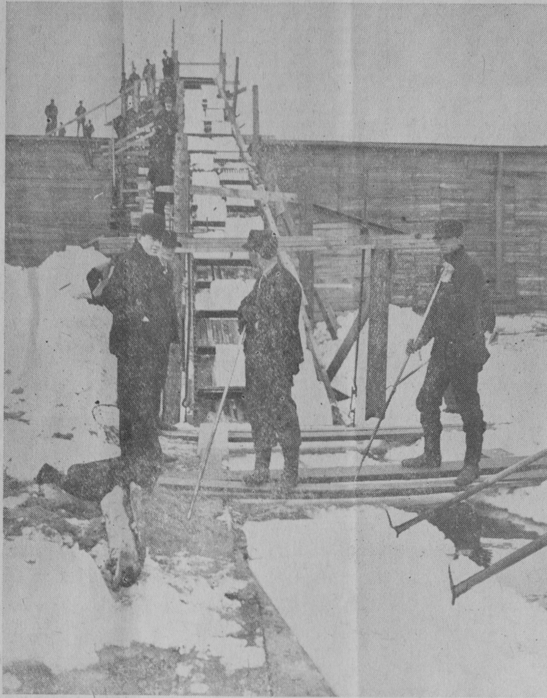
HARVESTING ICE was one of the important winter-time industries at East Tawas many years ago. Several hundred men were employed each winter in cutting, storing and shipping this product of nature. Large sheds were located on Tawas Point for storage of ice and one of these buildings is pictured above. A conveyor system is being used to move ice from the water to the building. Sawdust was used as an insulating material in storage. Large quantities of ice were used by the Detroit and Mackinac Railway Com-
