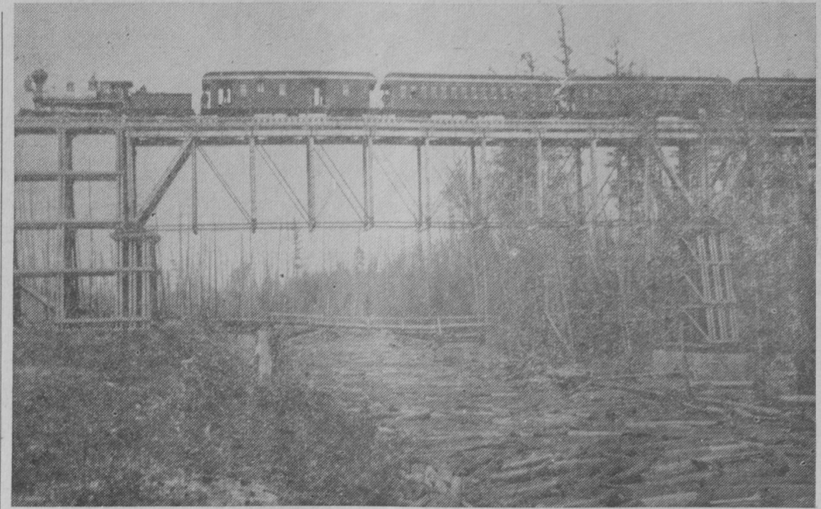
RIDING THE HIGH IRON over this wooden bridge which spanned the Rifle River is a locomotive and train of coaches of the Detroit, Bay City and Alpena Railroad Company, forerunner of the present-day Detroit and Mackinac. This bridge was completed in 1883 and its design was patterned after railroad bridge engineering developed during the Civil War. It was 75 feet above low water mark and was considered the highest railroad bridge in Michigan. Its total length was 986 feet, with two truss spans of 100 and 150 feet, being a combination of wood and iron. The rest of the length consisted of trestle work, containing more than a
