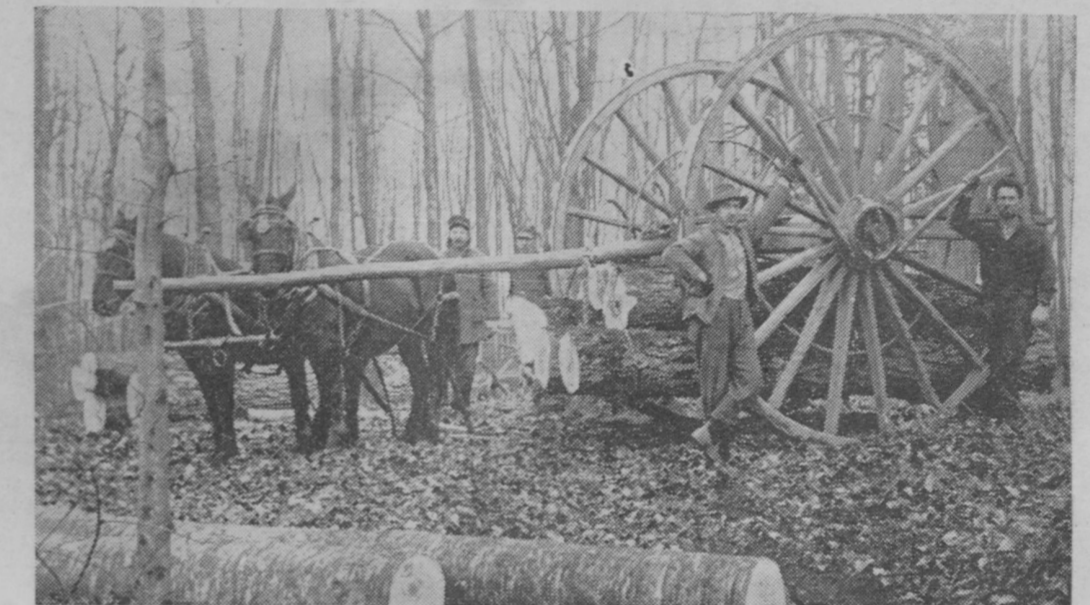
IN AREAS where there were no streams, huge wheels such as these were used to transport logs to the nearest river or railroad. Transportation of logs to the mill was a costly item in a lumber firm's operation.—Barkman Collection.
