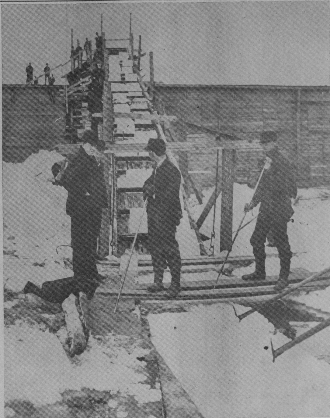
HARVESTING ICE was one of the important winter-time industries at East Tawas many years ago. Several hundred men were employed each winter in cutting, storing and shipping this product of nature. Large sheds were located on Tawas Bay for storage of ice and one of these buildings is pictured above. A conveyer system is being used to move ice from the water to the building. Sawdust was used as an insulating material in storage. Large quantities of ice were used by the Detroit and Mackinac Railway Com-
