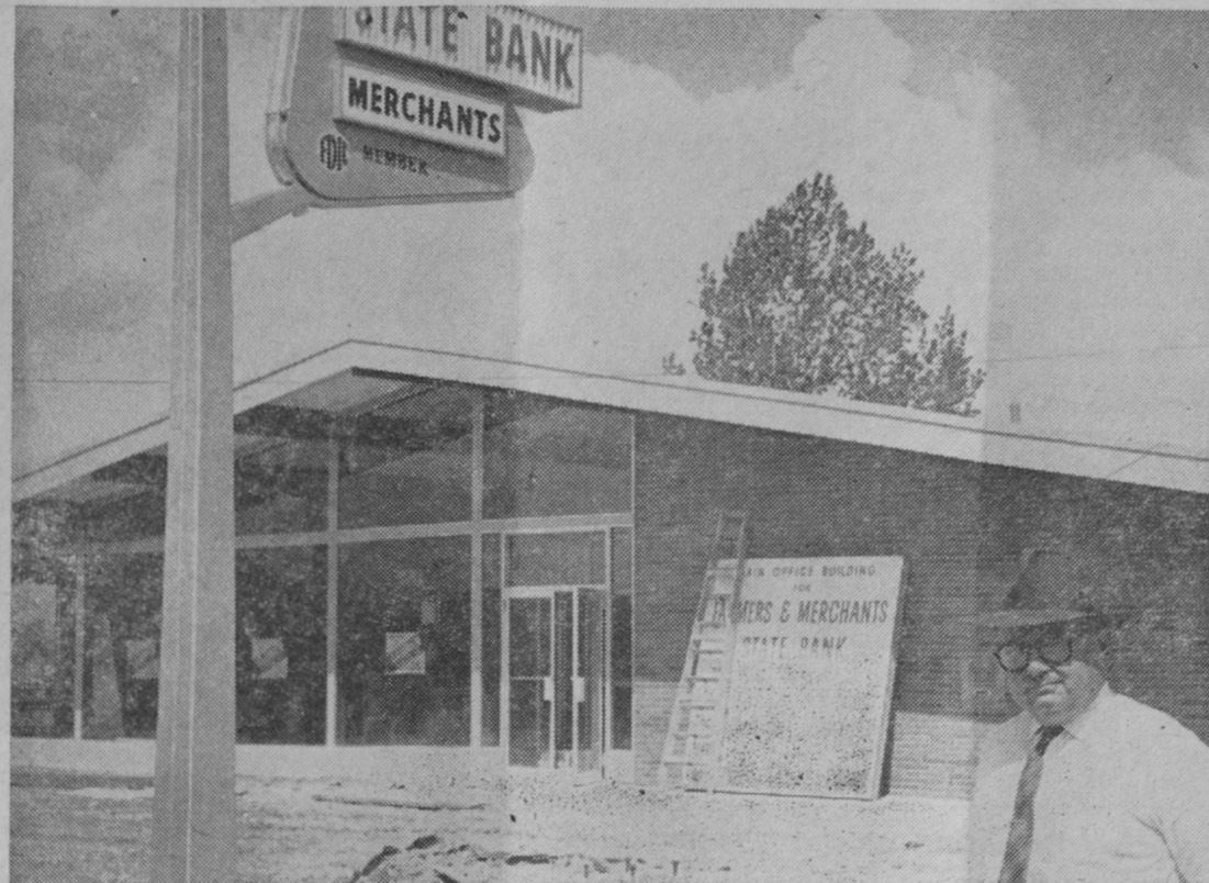
J. MORLEY STEVENSON, vice president and cashier of Farmers and Merchants State Bank, is shown at right standing in front of the bank's new main office at Hale. The general public is invited to attend an open house for the new building Tuesday, June 5. A ribbon cutting ceremony will be held at 9:00 a. m. that day. Business will be conducted in the new quarters starting May 28.—Tawas Herald Photo.
