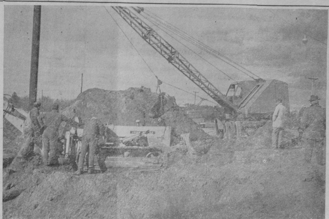
WORK started Monday morning on tunneling Park. This picture shows the city dragline with under M-55 for extension of sanitary sewer on Supt. Reginald Bublit standing second from right.—Tawas Herald Photo.
