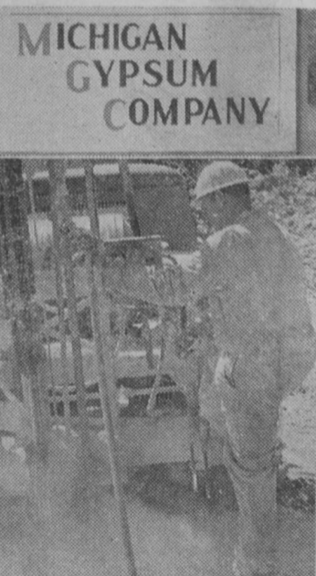
A ROTARY DRILL is pictured at left while Jack Thornton prepares to blast at center. Overall view of the crusher and stockpile area is shown at top right. A Detroit and Mackinac locomotive pulls a string of loaded gondola cars at lower right.—Tawas Herald Photos.
