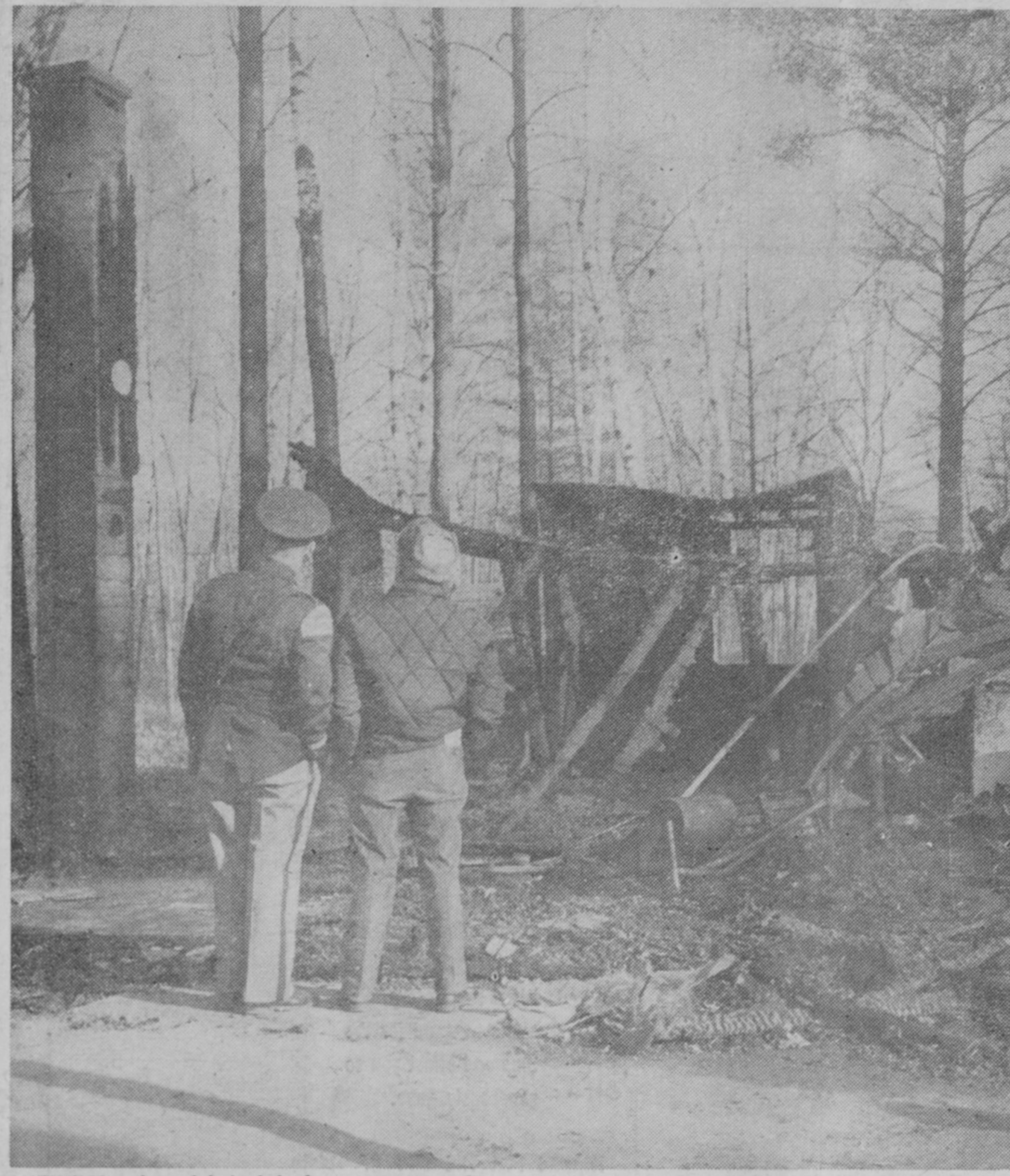
VIEWING the debris left from a cottage fire early Saturday morning in which a Wurtsmith Chief Robert Foster, left, and Fire Chief Howard Hofacer. Investigators said the blaze was caused by a faulty space heater.—Tawas Herald Photo.
