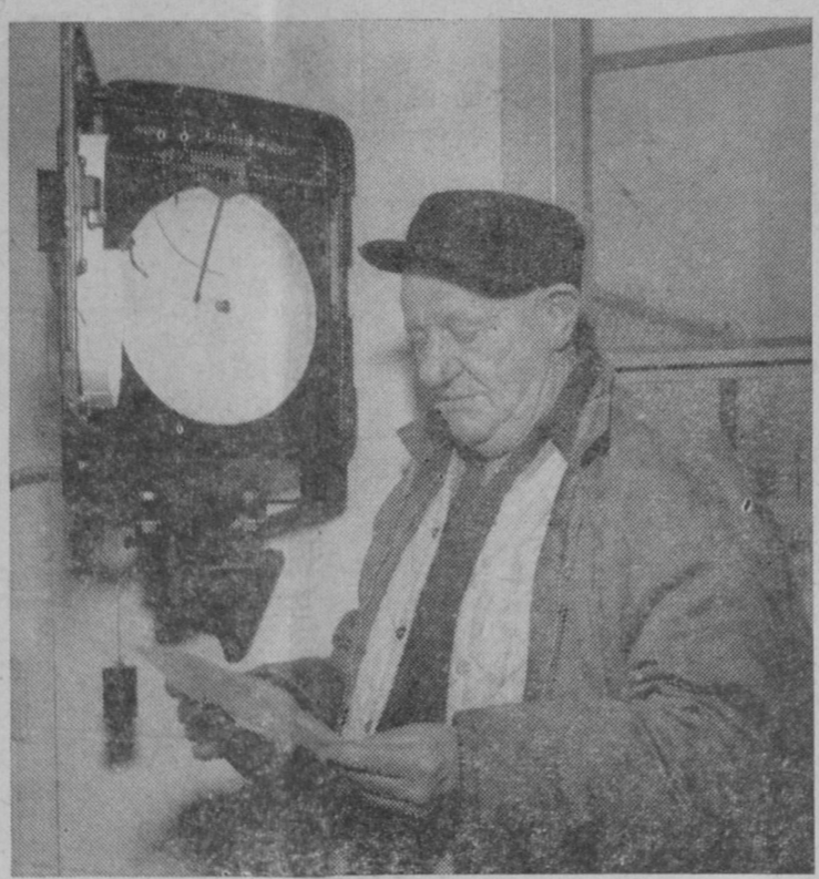
CHECKING ON pumpage at the city's disposal plant is Matthew Pfeiffer, veteran city foreman. The meter on the wall also shows if pumping stations are operating properly.—Herald Photo.
