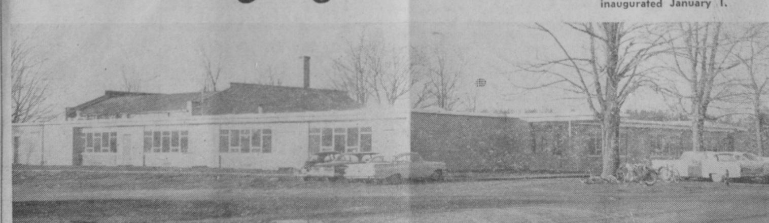
TAWAS AREA SCHOOL'S new Tawas City Elementary Unit was completed last fall. The structure is located on the site of the old frame school building. New classrooms were attached to the existing gymnasium and four-room unit. The new building now houses sections of kindergarten through four grades, all fifth, sixth and seventh grade students.
