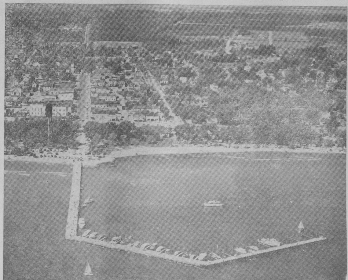
MICHIGAN WATERWAYS COMMISSION dock at East Tawas is shown in this aerial view. Tuesday morning's fire started mid-way on the "leg" extending out from Newman Street. The fire was stopped near the angle of the dock at lower left in this picture.
