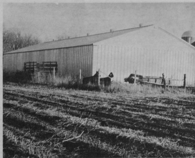
1960 — Built the large loose housing pole barn shown in the rear . . . the first step in a well-planned feeding and milking area.
