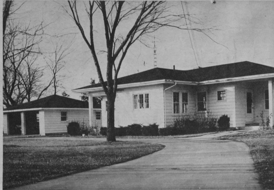
1954 — Tore down the old house that stood here and put up this attractive, modern farm house. Mrs. Knutson is the official bookkeeper.
