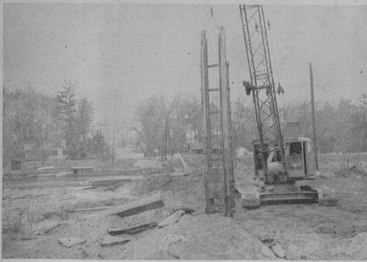
CONSTRUCTION has started on a new bridge to carry traffic over the AuSable River at Oscoda. This new structure is to replace an old one-lane bridge which was removed last winter. The dragline shown here is being used to construct footings for the new structure.—Tawas Herald Photo.
