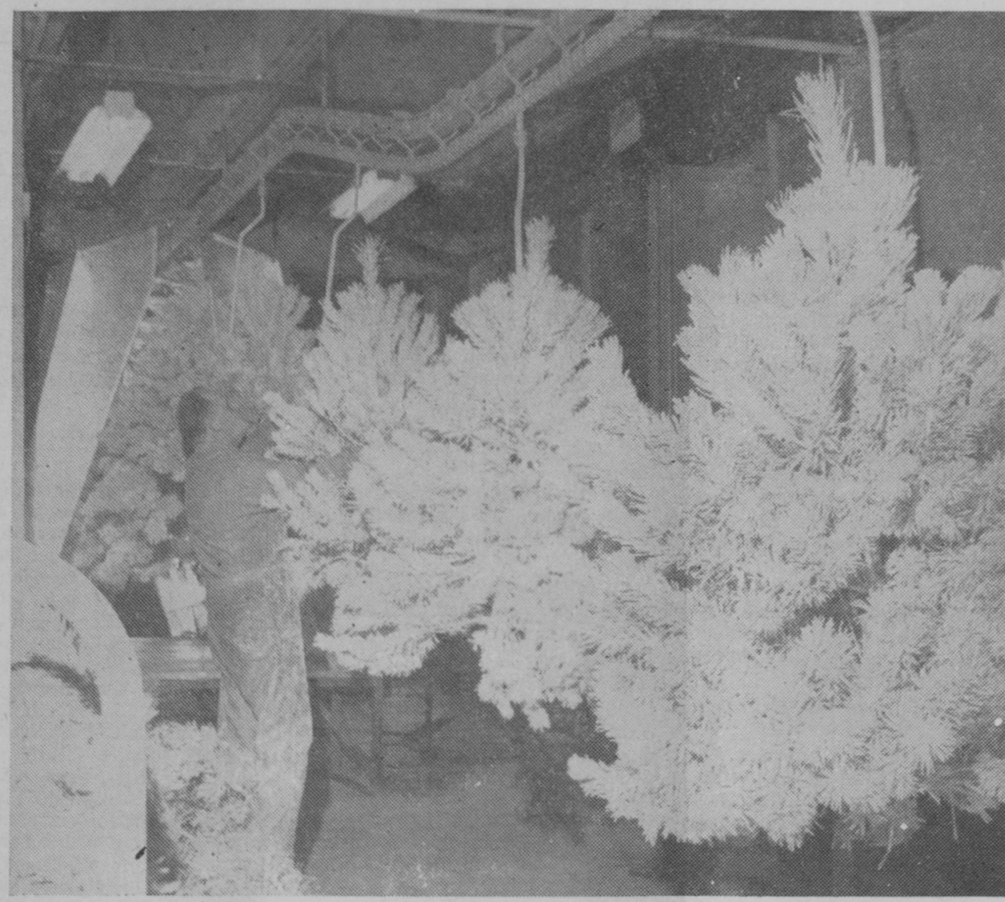
CHRISTMAS TREES sprayed with velvet are shown emerging from a drying oven at the plant of Creative Decor Products, Incorporated, East Tawas. Freshly cut trees are sprayed with rayon fiber using a special electrostatic process.—Tawas Herald Photo.
