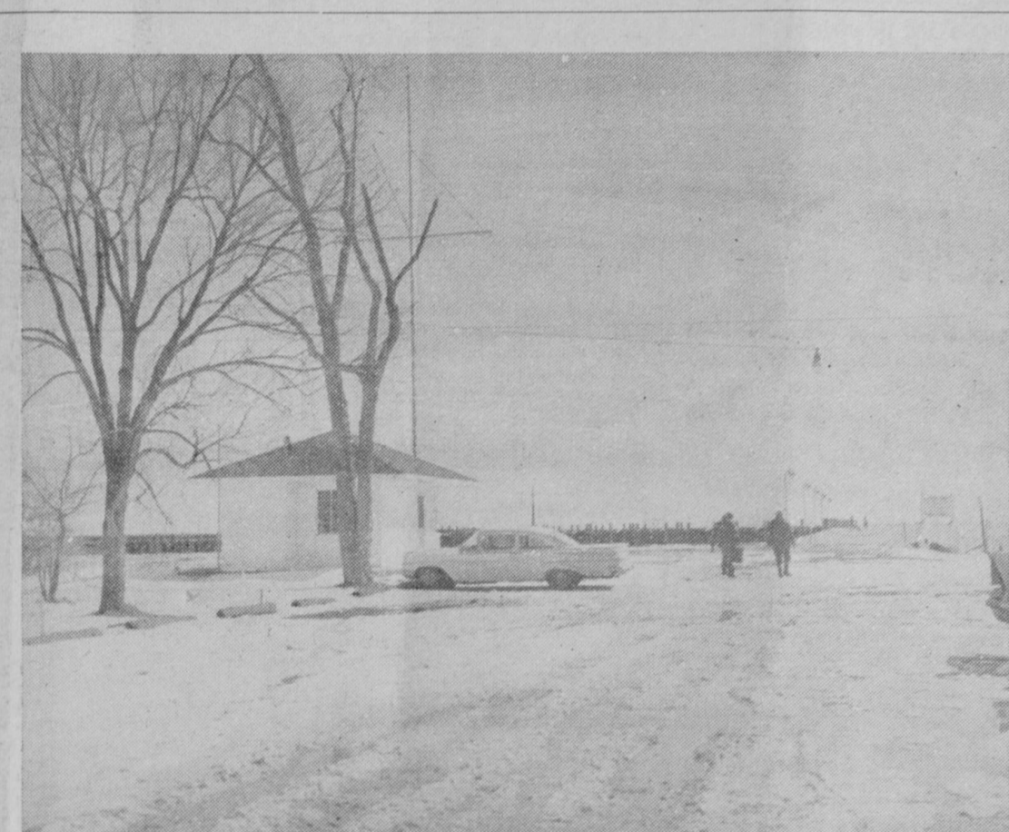
POSSIBLE SOLUTION to a parking problem at the state park in East Tawas may be reached this week. Tentative approval has been given for construction of a 60-car parking lot left of the harbormaster's office (above left), with a turning
