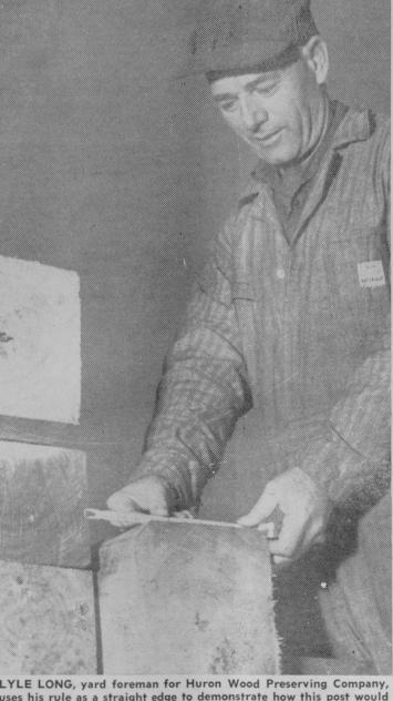
LYLE LONG, yard foreman for Huron Wood Preserving Company, uses his rule as a straight edge to demonstrate how this post would not meet state highway department specifications because of the beveled corner caused by removal of bark.—Tawas Herald Photo.
