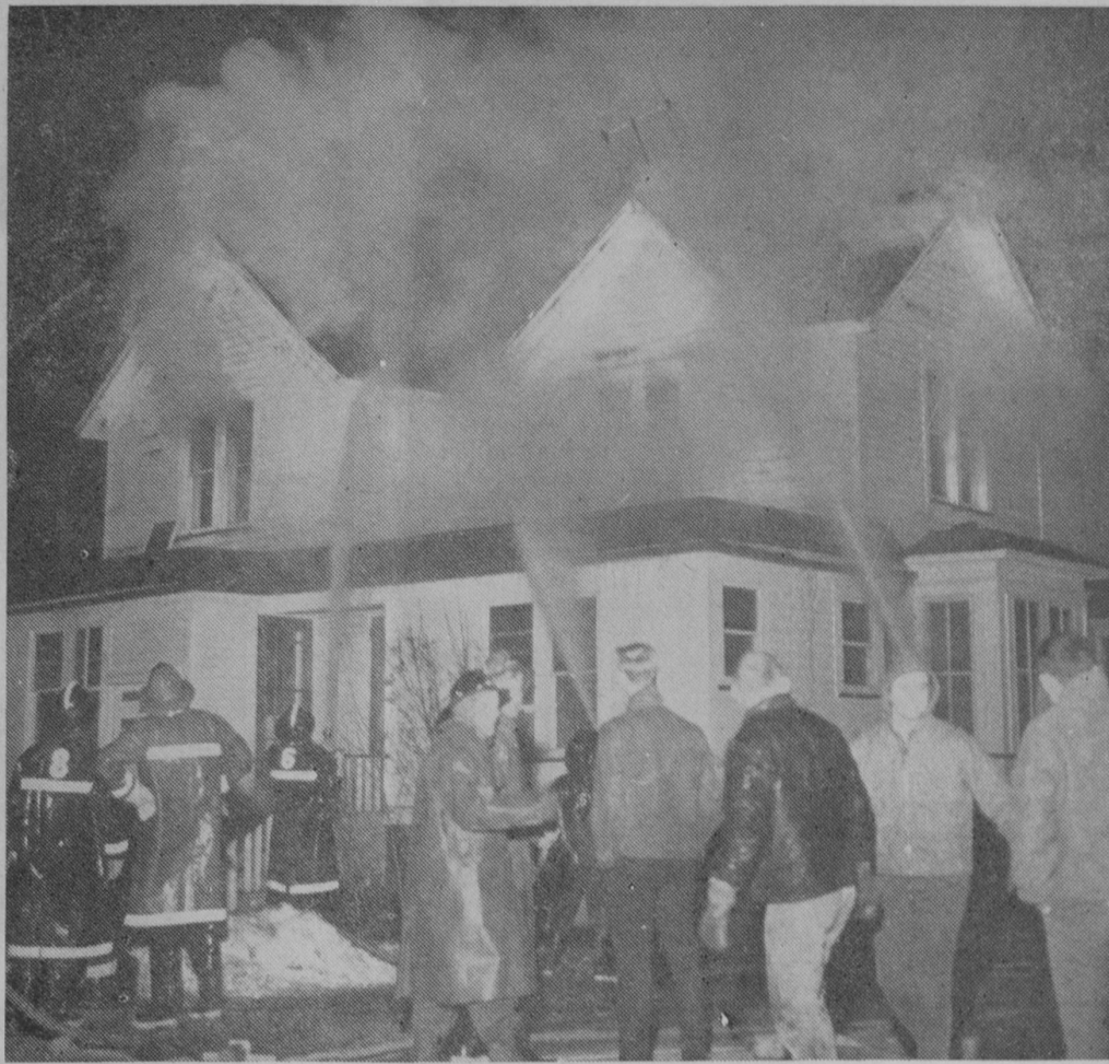
FIRE Sunday night and early Monday morning completely demolished the two-story home and office of Mrs. Zella Muilenburg, East Tawas chiropractor. Firemen from East Tawas and Tawas City battled the blaze for approximately eight hours. (See story on page 1.)—Tawas Herald Photo.
