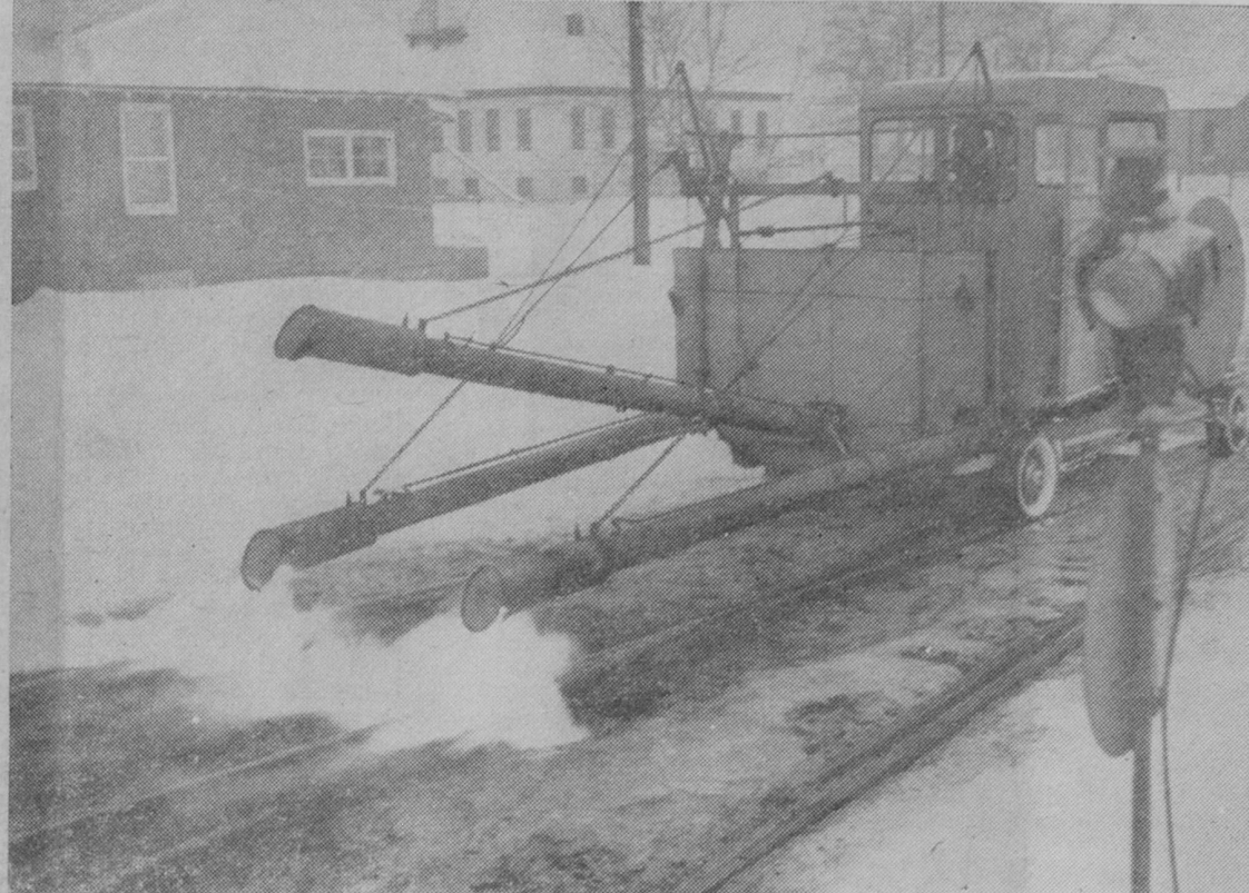
COLD WEATHER has forced the Detroit and Mackinac Railway to use drastic means to keep its crossings and switches free of ice. This unit, normally used to burn weeds along the roadbed, was melting ice Friday.—Tawas Herald Photo.
