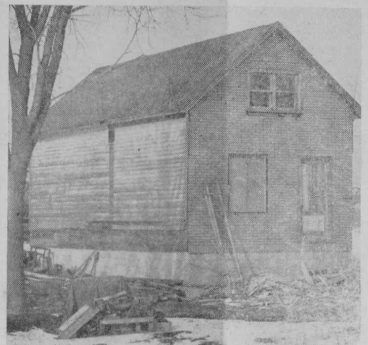
This old building proved a controversial subject in Tawas City.
