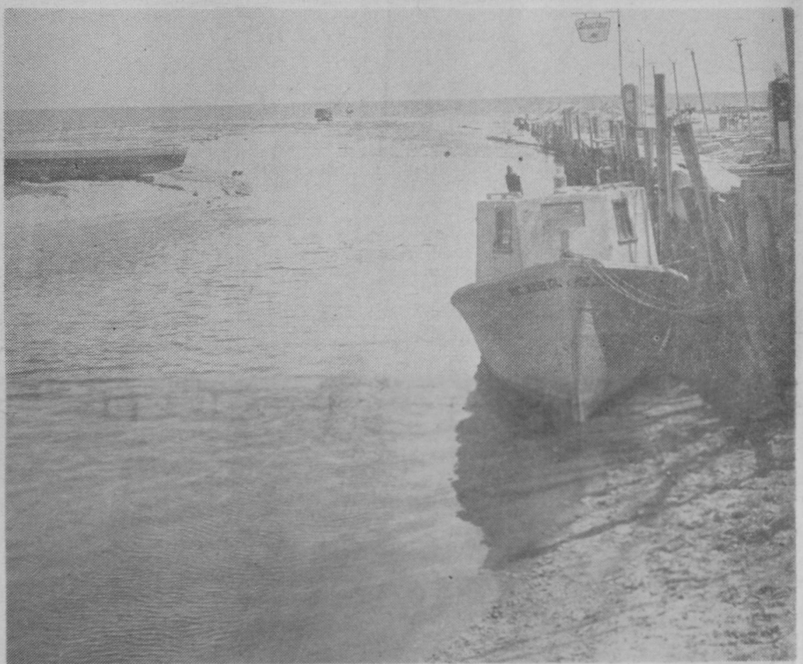
LOW WATER at the Tawas River mouth is shown in the above picture. Work was started Monday on dredging a channel 40 feet wide and about four feet deep to allow passage of small craft into Tawas Bay. A dragline is shown at top center cutting through a sandbar which blocked the river mouth. Contractor for the work was A. J. Merrill and the project was financed jointly by the City of Tawas City and local businessmen.—Tawas Herald Photo.
