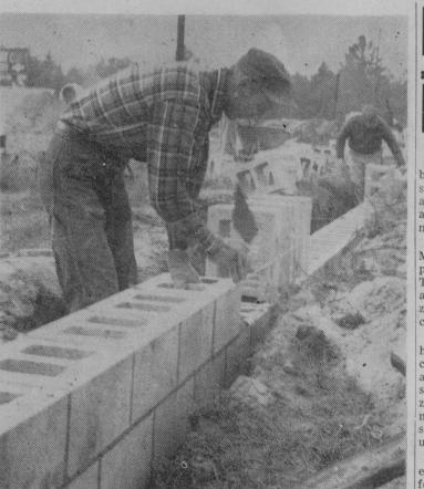
WORK has started on construction of a new plant to house Tawas Trailers, Incorporated, which was struck by fire last month. Workmen are shown above laying cement blocks for the new building, owned by Truman Barbier and located in Tawas Center on US-23. -Tawas Herald Photo.
