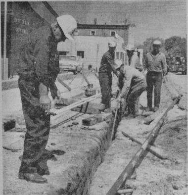
AN INSPECTOR EXAMINES the installation of a gas main in front of the East Tawas City Hall.
