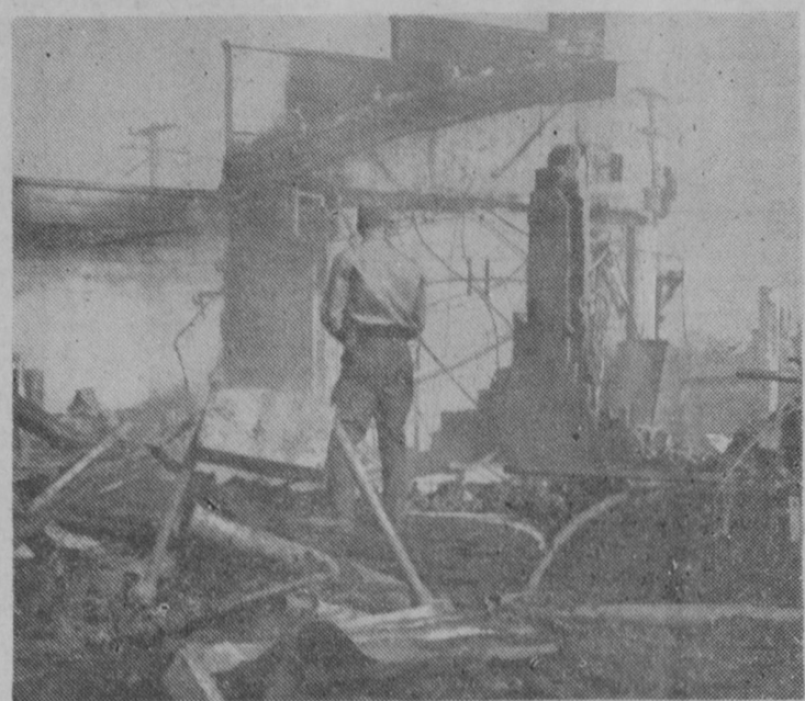
ONLY a shell filled with burned timbers and twisted metal remained after Tuesday morning's fire which swept Tawas Trailer, Incorporated, plant at East Tawas.
