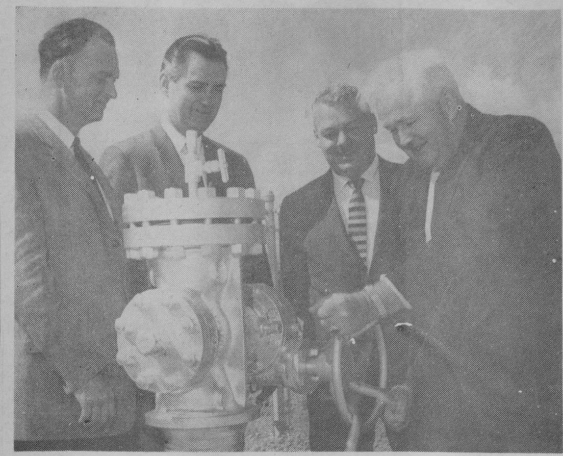
NATURAL GAS was turned into mains of Michigan Consolidated Gas Company last Wednesday morning commencing service to the Tawas. Watching Chamber of Commerce President Ralph Western turn the valve to officially open
