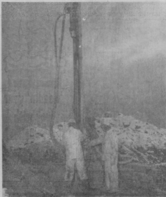
DRILLING through 31 feet of limestone rock at Whitestone Point is this equipment of Power Blasting Company, Incorporated, explosives engineers, Oak Park. Explosives will be placed in the drill holes for blasting the rock.—Tawas Herald Photo.
