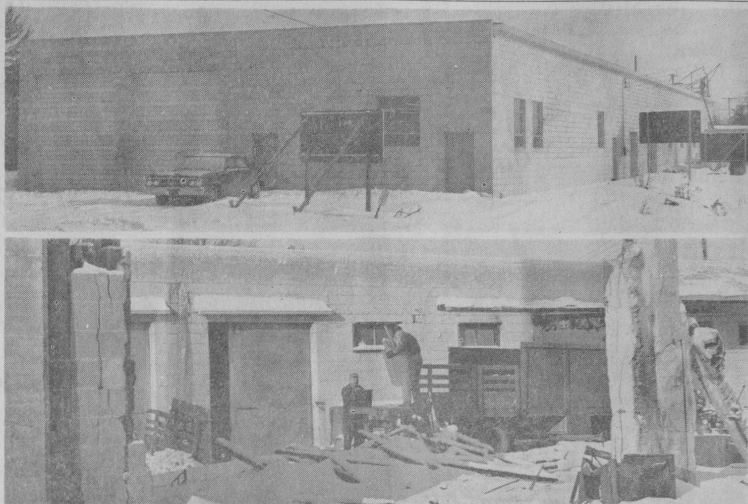
NEW HOME of Tawas Trailers, Incorporated, is pictured at top as workmen were putting the finishing touches on the roof. Framed by ruins of the old Anderson Coach plant, the lower picture shows a truck being loaded with equipment from a warehouse which quartered the trailer firm temporarily since a fire last October. —Tawas Herald Photos.
