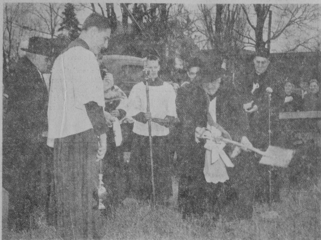
CONSTRUCTION of a new church for St. Joseph Parish was one of the accomplishments of the Rev. Fr. Robert Neuman during his 22 years as priest at the East Tawas church. He is shown here during 1952 ground-breaking ceremonies for the new church.—Tawas Herald Photo.
