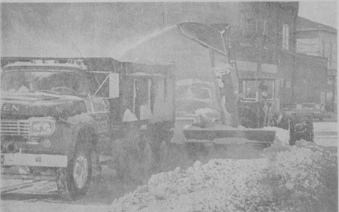
EAST TAWAS' new snow blower had its first real test last Thursday and it passed with flying colors. Supt. of Public Works Paul Ropert said that snow removal was speeded greatly through
