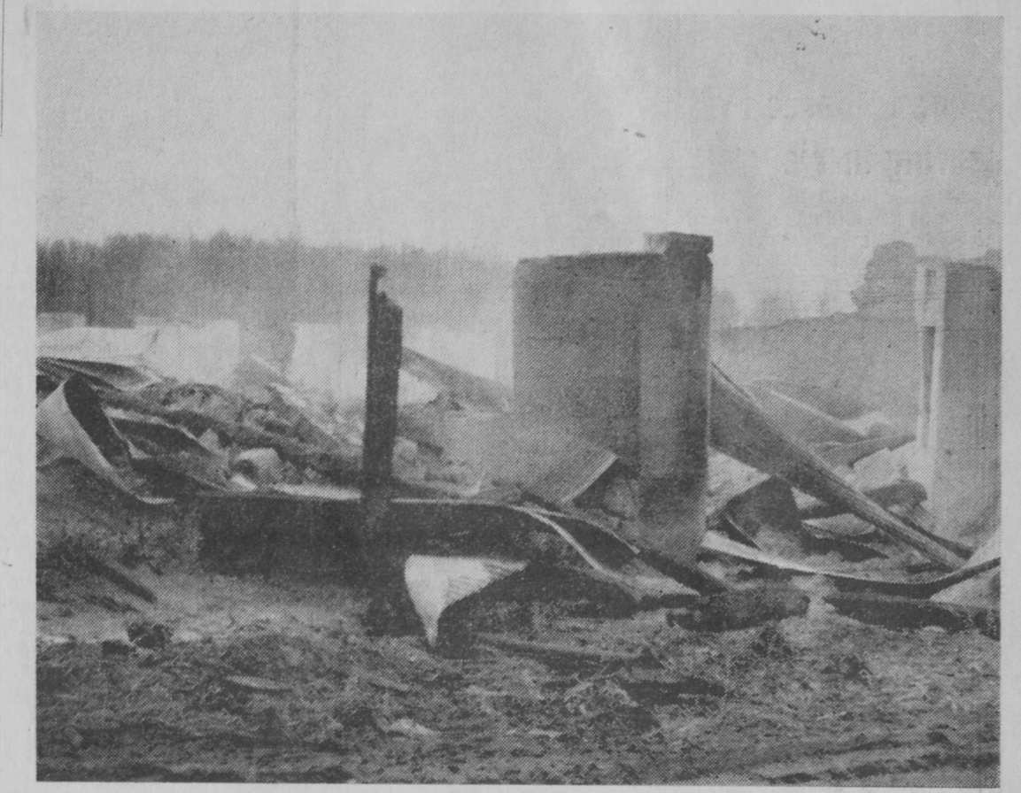
ONLY thing remaining of George Waters' barn after a fire last week was the foundation pictured here. The blaze was out of control by the time it was discovered and the owner raced through the lower floor releasing cattle. Twenty calves and a cow were lost.—Tawas Herald Photo.
