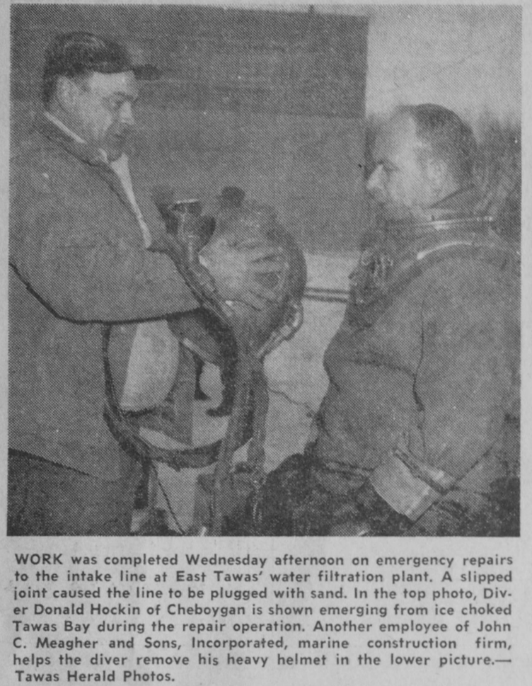
WORK was completed Wednesday afternoon on emergency repairs to the intake line at East Tawas' water filtration plant. A slipped joint caused the line to be plugged with sand. In the top photo, Diver Donald Hocking of Cheboygan is shown emerging from ice chocked Tawas Bay during the reboyan operation. Another employee of John C. Meagher and Sons, Incorporated, marine construction firm, helps the diver remove his heavy helmet in the lower picture.—Tawas Herald Photos.
