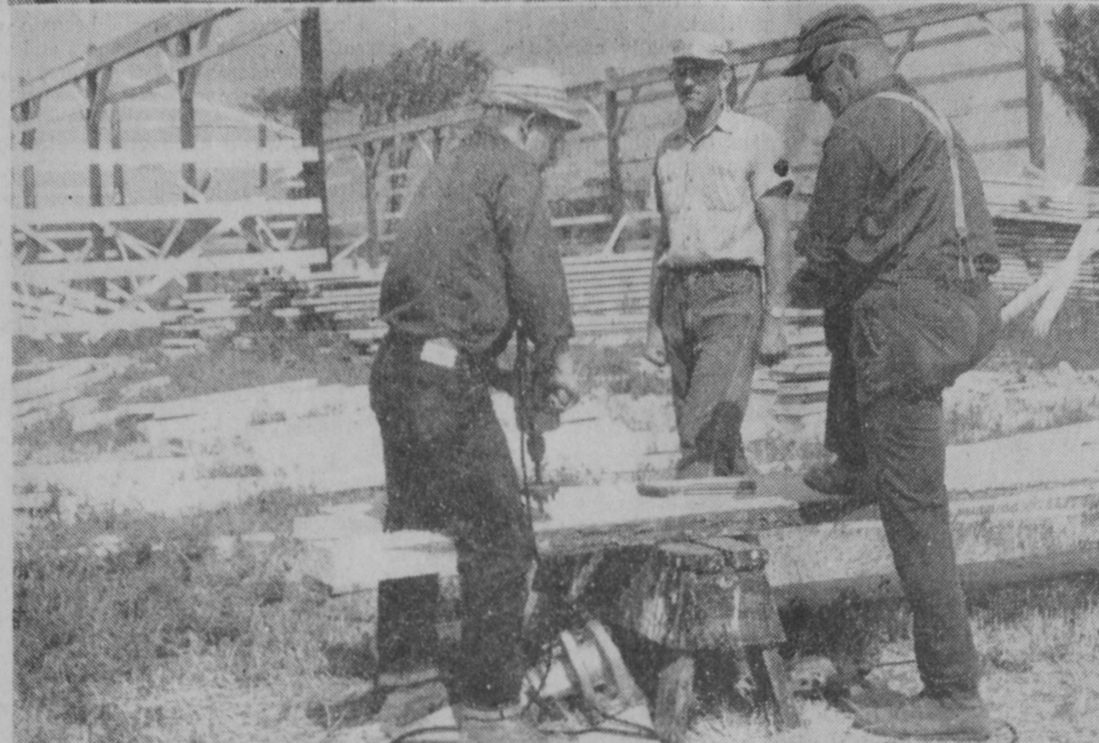
NEW BARN —Leonard Robinson, Reno Township, is now in the process of building a new barn at his farm located five miles south of Hale on M-55. Barn construction is something rather scarce in these days of high costs and Robinson is building a 96 by 56 pole-type structure to house cattle, hay and machines. The oak timber being used in construction was cut and sawed into lumber from his own woodlot. Robinson is shown in the top picture with the barn in the background. In the lower picture, he talks with Paul Meiser of Prescott and David Clayton of West Branch, who are assembling rafters.—Tawas Herald Photos.
