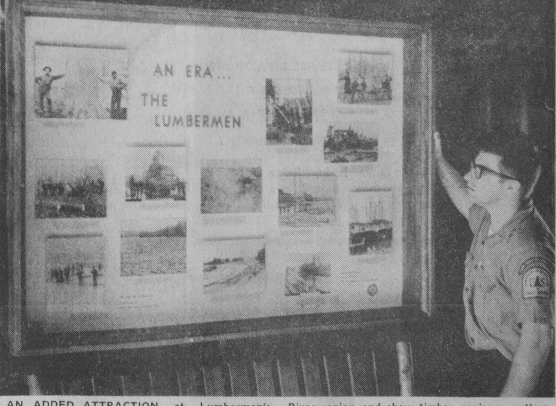
AN ADDED ATTRACTION at Lumbermen's Monument is a new historical display installed Friday in the comfort station by the United States Forest Service. Tawas District Ranger Loren Woerpel is shown looking over a display case containing a collection from the lumbering days. The pictures, furnished by The Tawas Herald, depict logging operations in the AuSable River region and show timber cruisers, cutters, rivermen, methods of transportation and mills. Each picture is individually captioned with a brief explanation. The case was constructed by John Ristow of the forest service and Woerpel designed the picture arrangement.—Tawas Herald Photo.
