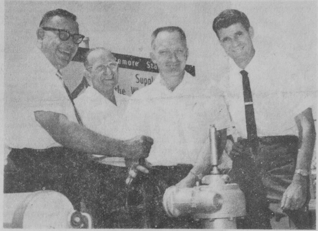
MARKING a historic moment in the progress of Isosco County, natural gas was turned on Tuesday for the first time to serve Hale. Key figures in attending the ceremony were, from left: James Preston, district manager, Michigan Consolidated Gas Company; D. D. Preussall, Hale businessman; Lyle Bernard, Plainfield Township trustee, and William Smith, Tawas area manager for the gas company.—Tawas Herald Photo.
