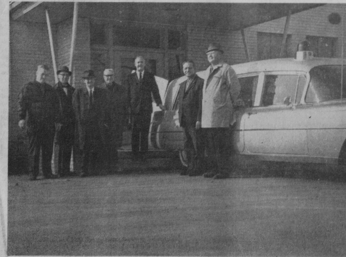
MEMBERS of the Tawas Hospital Board are shown above inspecting new blacktop at the hospital's emergency entrance. This project, part of a three-phase undertaking to complete paving at the hospital, was underwritten by a benefit dinner dance last September which netted $1,000. An additional $550 was borrowed for the project, which is to be paid off by hospital me-
