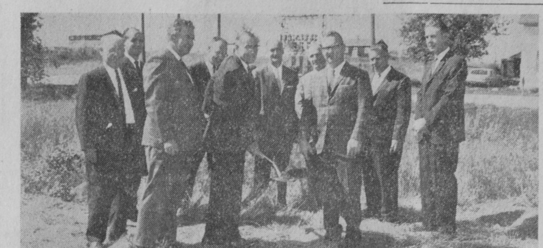
GROUND was broken last week for Consumers Power Company's new Rose City area service center. Louis A. Vaupre, Bay City Division manager, assisted by a number of representatives of Rose City area community groups, is turning over the first shovel of earth. The facility will be work center for about 30 CP employees, including some now stationed at Mio, Hale and West Branch.
