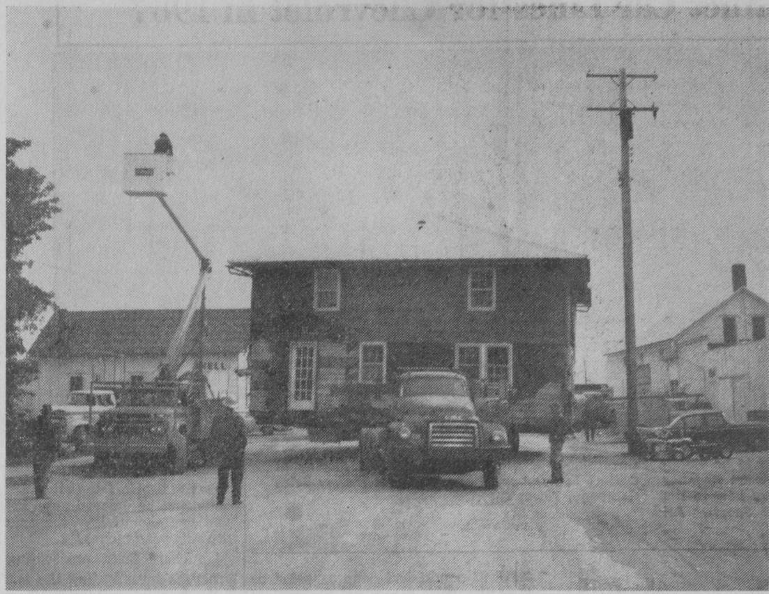
MOVING DAY for this old residential building was last Tuesday at Hale. Forward Oil Company is in the process of clearing the northwest corner of the M-65 intersection for a new super service station and this building was moved to a new location near the Methodist Church. Crews of Michigan Bell Telephone Company and Consumers Power Company were on hand to splice telephone and power cables during the all-day project. The building once served as quarters for the A. E. Greve Drug Store and telephone office and later as a residence. The old township hall, which was converted years ago into a service station, is also to be removed.—Photo by Ira Scofield.
