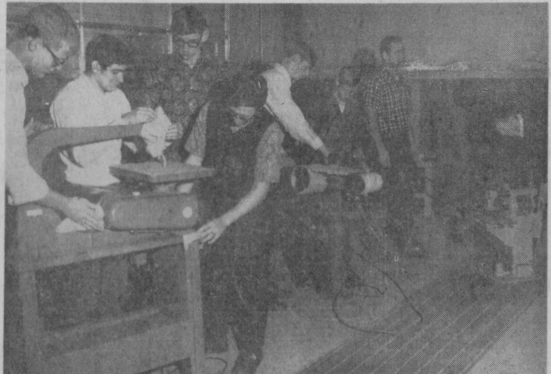
EQUIPMENT is now being readied for placement in the new metal shop at Tawas Area High School. This picture shows Robert Reasner, instructor, second from right, supervising the cleaning and painting of machines. The school
