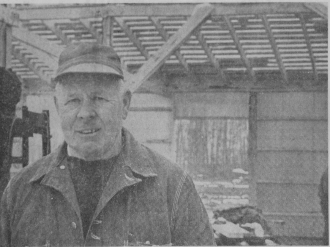
FIVE YEARS AGO, April 1, 1962, the mill of Hale Wood Products was destroyed by fire. As workmen began rebuilding the mill and salvaging equipment damaged by the flames.—Owner Albert Gardner was pictured at the time. Herald Photo.
