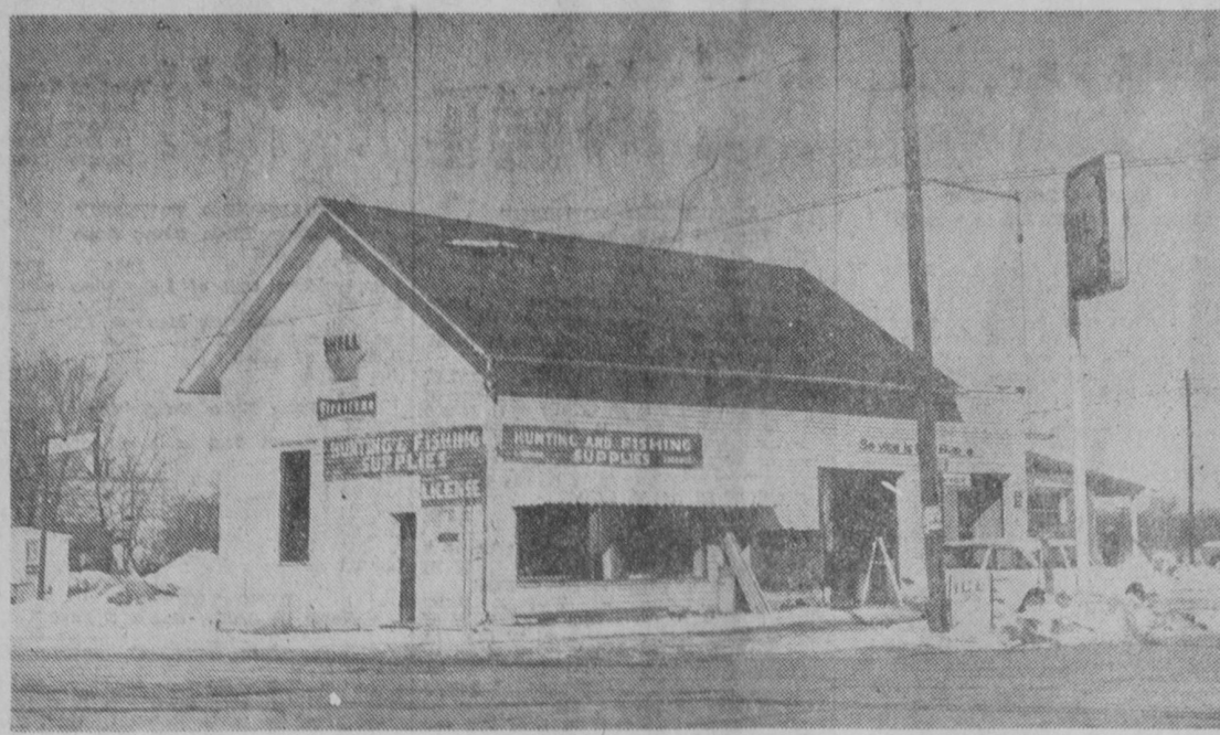
WORK STARTED last week on removing this old building at Hale. Used as a gasoline service station in recent years, it was once the Plainfield Township Hall. Forward Oil Company has constructed a modern new service station to the right (north) of the building and the move into these quarters was completed about two weeks ago.—Tawas Herald Photo.
