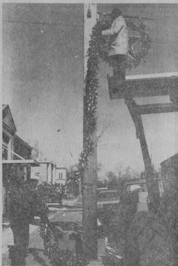
CITY CREWS were busy last week installing Christmas street decorations at East Tawas. City Foreman Edward Lixey tosses a band of colored tinsel to the workmen perched on the tractor bucket during decoration of a power pole at the Newman-State Street intersection.—Tawas Herald Photo.
