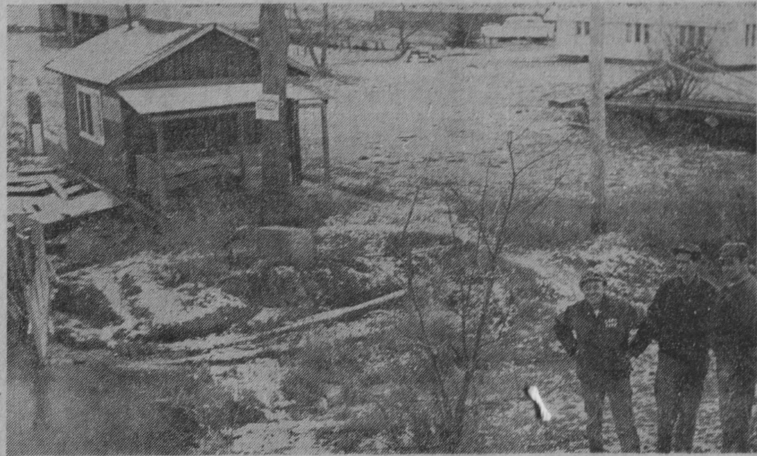
WEST SIDE of the Tawas River mouth has been sold and is to be developed into a new charter boat marina. The sale included a tackle shop at left, boat sheds and harbor in the background and the home at right which is to be converted into a restaurant.—Tawas Herald Photo.
