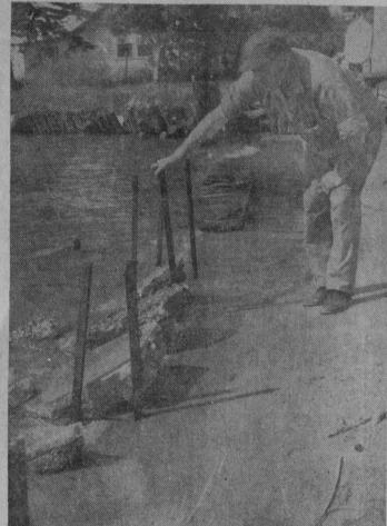
CITY FOREMAN Arthur Wegner inspects a section of sanitary sewer which buckled last week. Located along the shore, water washed under the main and caused trouble.-Herald Photo.
