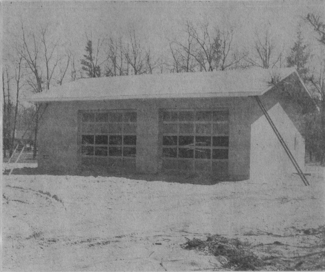
MEMBERS of Grant Township Fire Department held their first meeting Monday night in the new fire hall at Sand Lake. The building, financed by a special vote of the people and through volunteer efforts of firemen, was completed last week. The department received delivery on its first fire-fighting unit this week and expect to place an order for a larger truck and pumper in the near future.—Tawas Herald Photo.
