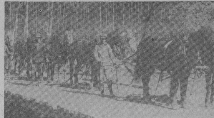
A HEAVY TRANSFORMER was moved from the railroad station at Hale to Cooke Dam with the aid of several teams of horses.
