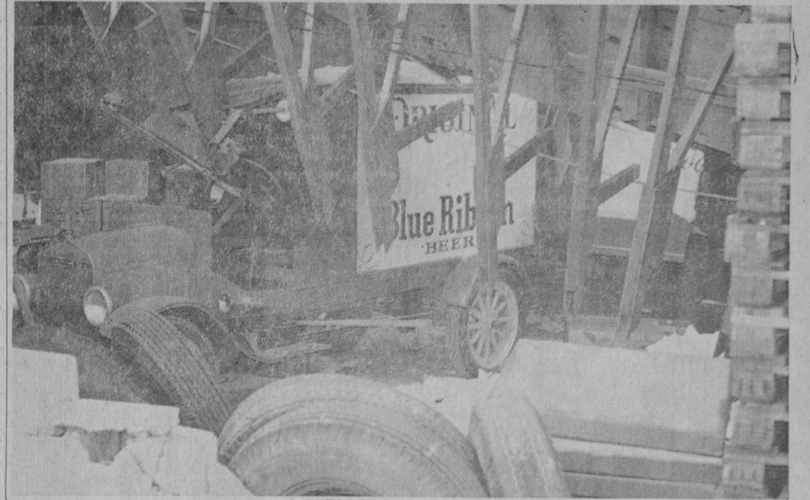
DAMAGED December 31 when Grabow Distributing's warehouse collapsed at National City was this old Model T Ford truck owned by Grabow. The truck was used for promotional activities. Part of the roof can be seen hanging down into the building.—Tawas Herald Photo.
