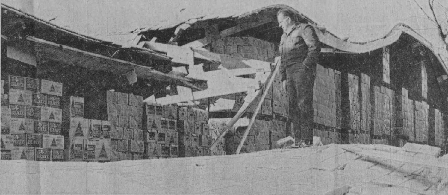
A COMBINATION of snow and high wind last Tuesday morning caused Grabow Distributing's warehouse to collapse at National City. No one was in the building at the time. Carl Grabow stands on one of the collapsed walls while he surveys a large quantity of beer which had to be moved into storage at Whittemore. George
