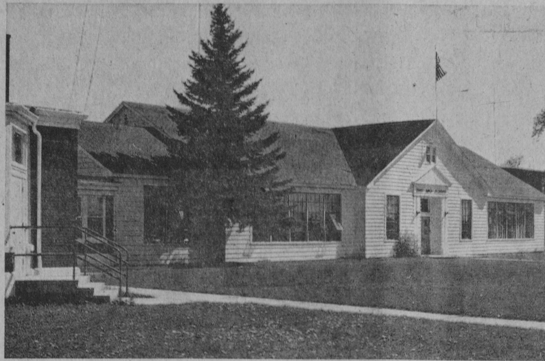
ON JUNE 9, voters of Hale Area School District will decide on a proposal to replace the center wooden structure (above) with a new junior and senior high school building. The brick wing at left would be retained for elementary use, as would the gymnasium at far right.—Tawas Herald Photo.
