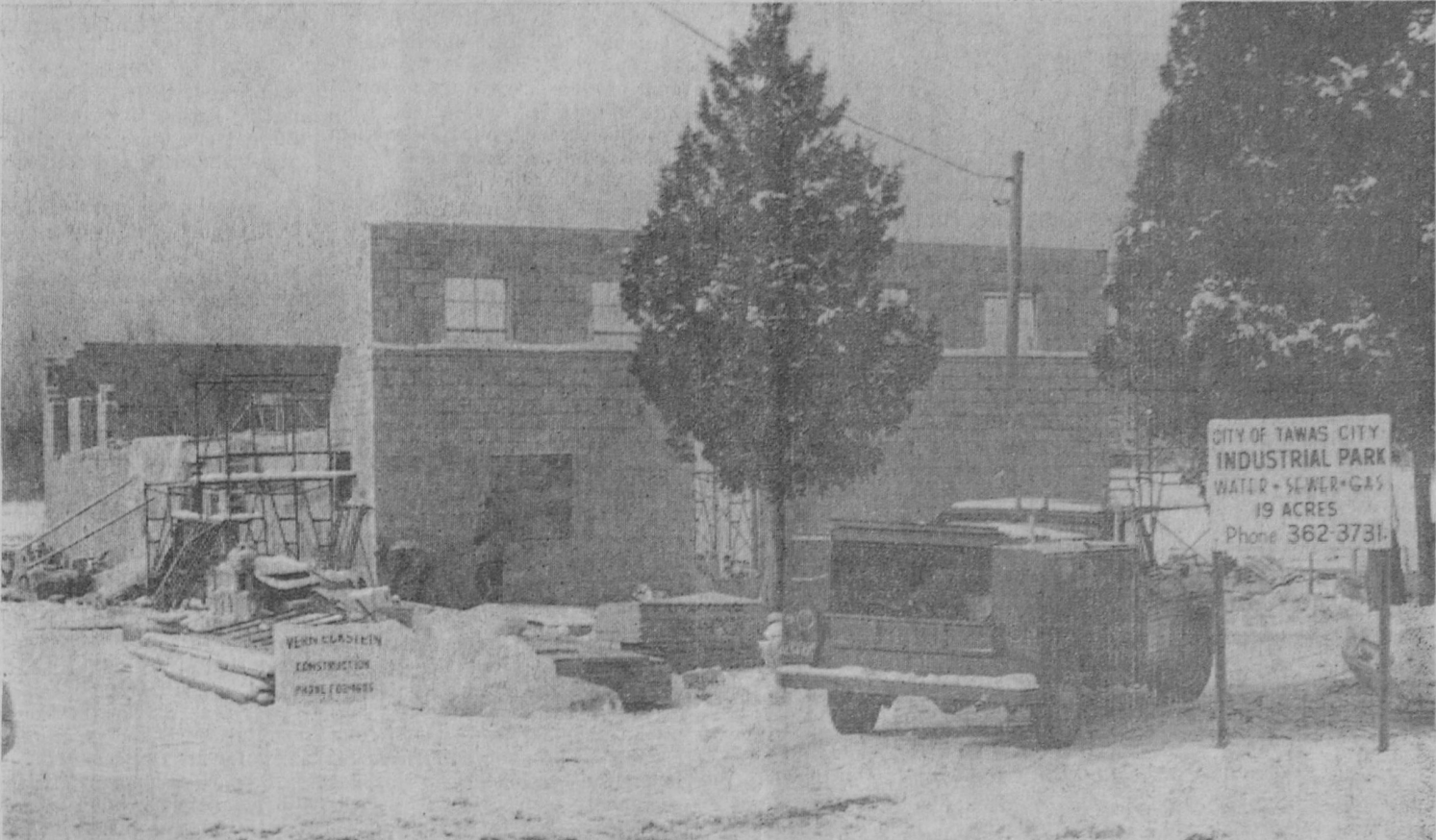
WORK on the new building to house Maher Pattern and Manufacturing Company's new plant on Ninth Avenue, Tawas City, looked like this Saturday morning. Construction started two weeks ago.—Tawas Herald Photo.
